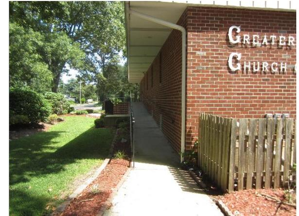
A rain garden can be implemented adjacent to the shed to the southeast by redirecting its downspouts into it to capture its runoff. A rainwater harvesting system can be implemented next to the southeastern corner of the building to manage even more stormwater from the rooftop. A preliminary soil assessment suggests that the soils have suitable drainage characteristics for green infrastructure.
