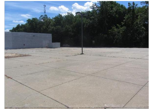
The large paved area alongside the Staples can be depaved or replaced with porous pavement. This area can potentially be used to manage additional runoff from the rooftop or parking lot. A preliminary soil assessment suggests that the soils have suitable drainage characteristics for green infrastructure.
