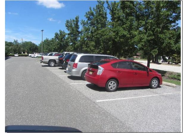
Parking spaces located on the southern end of the parking lot can be replaced with porous asphalt to capture and infiltrate stormwater. The parking lot slopes towards this end which would allow these spaces to manage stormwater generated from a portion of the parking lot and rooftop. A preliminary soil assessment suggests that the soils have suitable drainage characteristics for green infrastructure.
