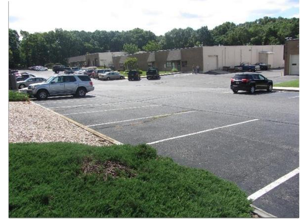
A bioretention system can be implemented in front of the building to manage stormwater from the parking lot. A trench drain can be used to direct the runoff into the bioretention system. A preliminary soil assessment suggests that the soils have suitable drainage characteristics for green infrastructure.
