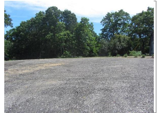
Portions of the damaged parking lot can be replaced with porous asphalt to capture and infiltrate a large portion of stormwater generated by the rooftop and pavement on the site. A rain garden can also be implemented near the entrance of the church to capture additional runoff from the rooftop and add aesthetic value. A preliminary soil assessment suggests that the soils have suitable drainage characteristics for green infrastructure.
